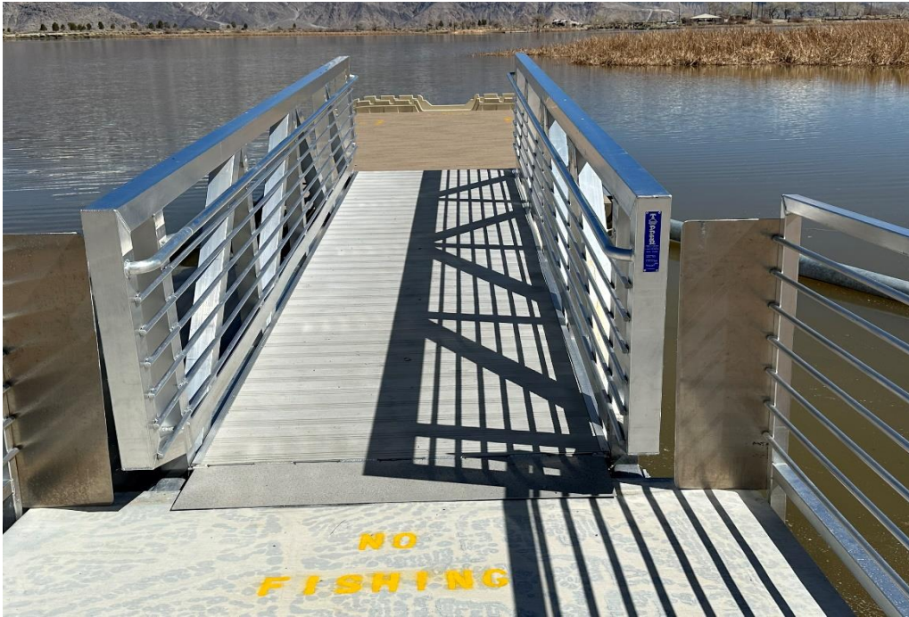
Gangway access onto the Boarding Float
